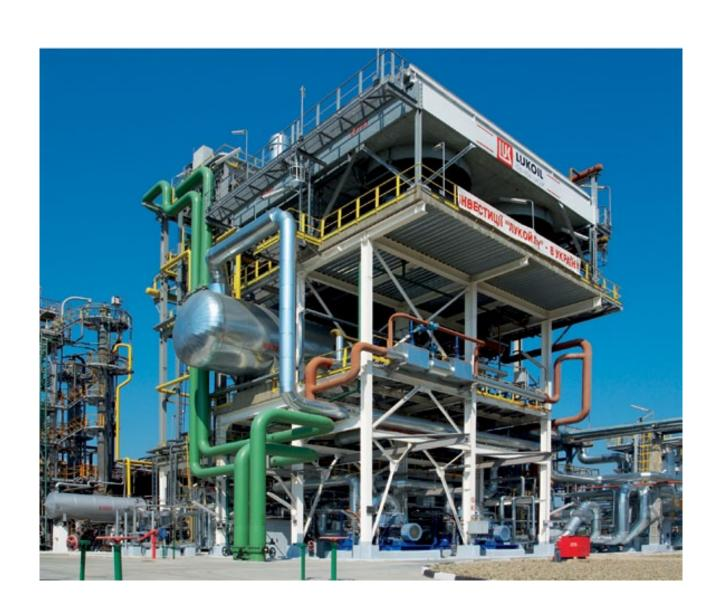
technology. Annual capacity of the new unit will be 182,000 tonnes of gaseous chlorine and 200,000 tonnes of caustic soda. The new capacities will enable Karpatneftekhim to produce caustic soda, which meets international quality standards, and to fully provide the plant's own chlorine needs. Commissioning of the unit is scheduled for the end of 2009.
